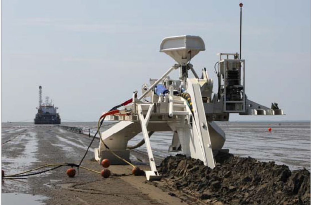
Plate 4-10: Example of a non-displacement plough (Source: Equinor)
