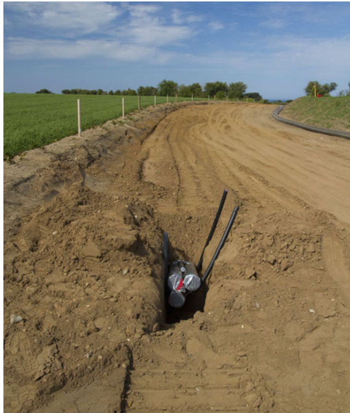
Plate 4-22: Example of backfilled trench following duct installation. End of duct visible in foreground awaiting joint bay construction and cable pulling (Source: Equinor)
