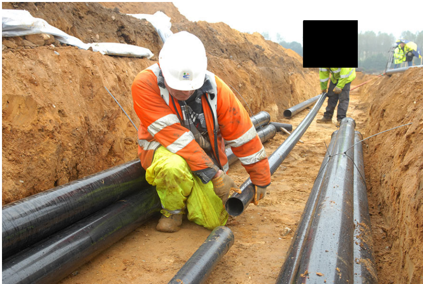
Plate 4-20: Example of hand laying ducts within open trench (Source: Equinor)
