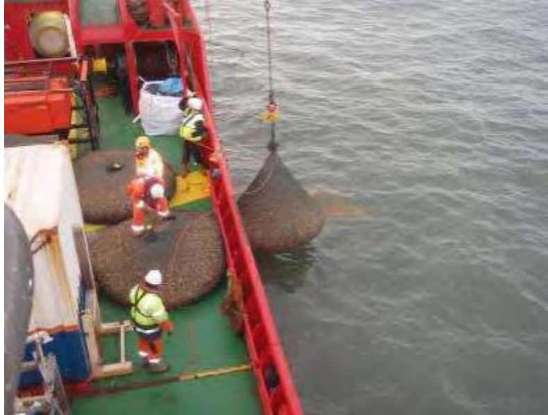
Plate 4-15: Rock bag installation (Source: Equinor)
